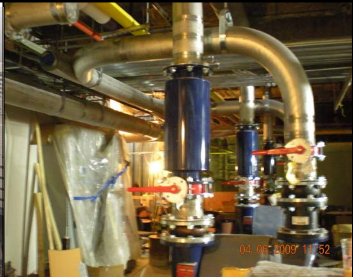
Pre-fabricated piping assemblies are installed on the job site.
