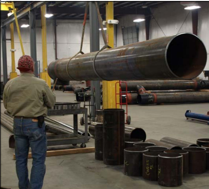
Condenser water piping is prepared for the plasma cutter.
