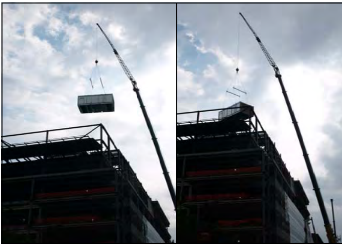
Installation of rooftop cooling towers high atop 650 Kendall
