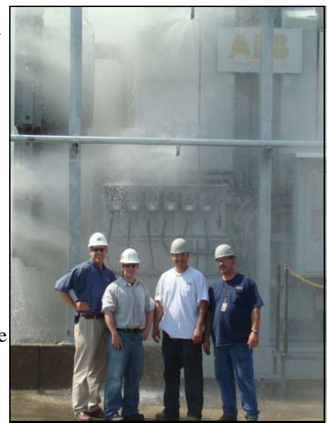
Chip Maurer, Brian Baima, Jose Diaz & Mark Dion at the Sandy Pond facility.
