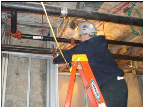
JCC Pipefitter Duncan MacLeod demolishes HWS/R
